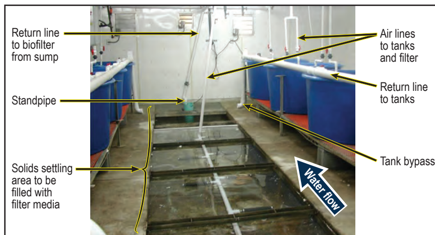
Figure 9. This waste pit and solids settling configuration shows select components and the water and air flow.
