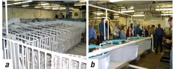
Figure 1. This unused swine barn (a) was converted into an active aquaculture facility (b).
