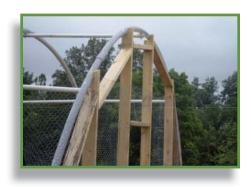
the vertical studs about 40 inches from the bottom. After the framing is complete, cover the ends with poultry wire. Drill 2½-inch holes in the base of each end frame, and drive the rebar (short for "reinforced bar") through the hole to secure the end in place. Additional bracing may be needed to help stabilize the structure during high winds and snow.
