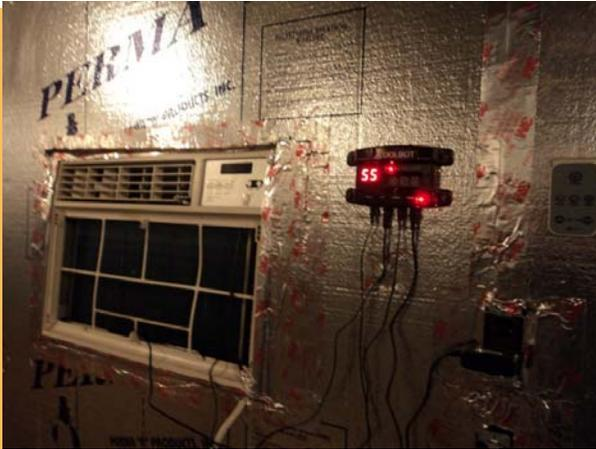
*CoolBot™ system hooked up to an AC unit in the Cold room (top). The CoolBot™ unit displaying the temperature inside the room (right).*
